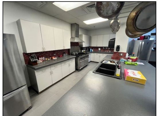
Station 154 counter top refinish
