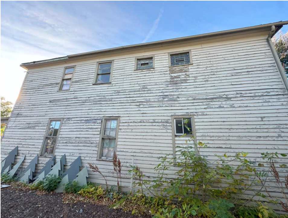
Figure 4: Existing North Elevation
