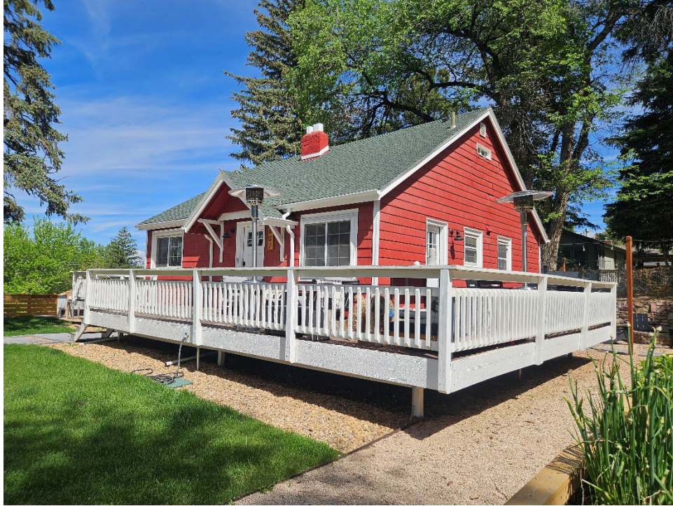
Primary (south) and east elevations of the residence, view northwest (Roll 26-450, image 103222; Emily Wren; 5/22/2026)
