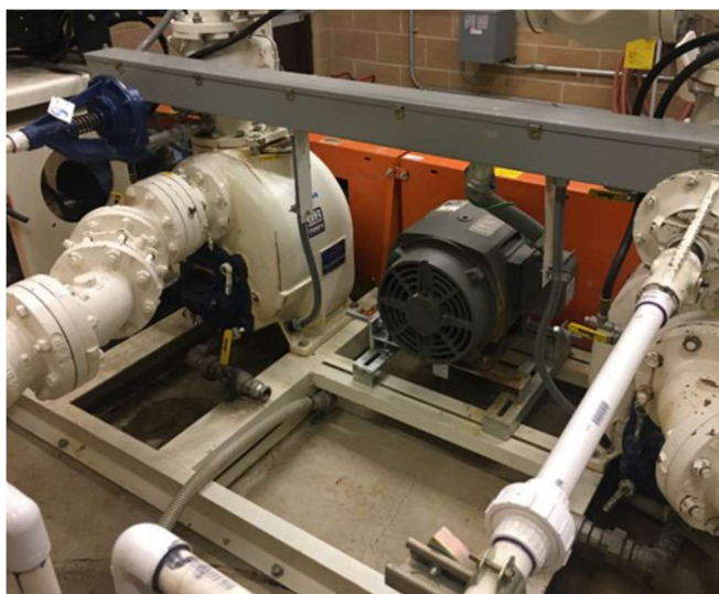
Old pumps at the Mitchell Creek Lift Station were replaced with new Gorman Rupp pumps.
