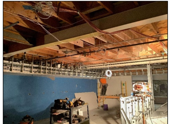
Douglas County High School remodel
