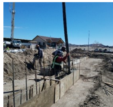
Concrete placed for new building foundation.
