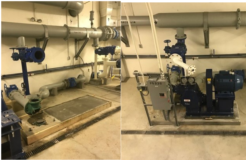
Plant Maintenance staff replaced the Mitchell Creek Lift Station pump 2 which will allow for more efficient pumping operations at the station.
