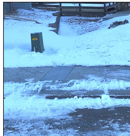
A chase drain clogged with ice buildup during the deep freeze of January.
