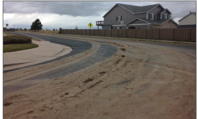
Heavy tracking onto a public road. This site inspection resulted in a notice of violation and cleanup order.
