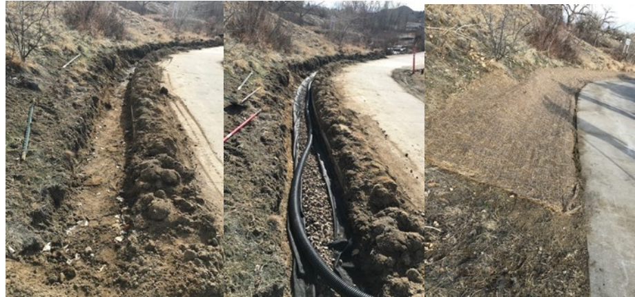
The Stormwater team installed an underdrain to keep ice off the Plum Creek trail
