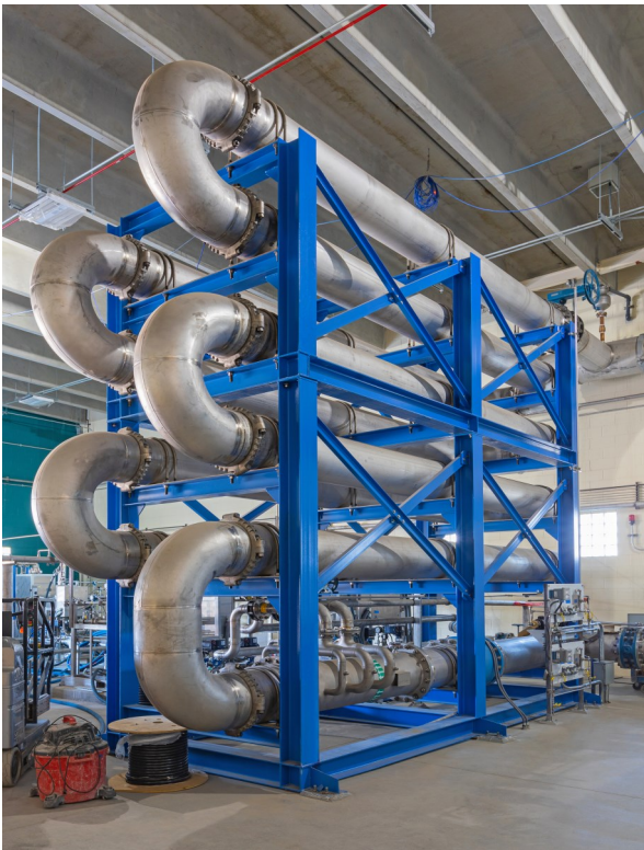
Stainless steel loop reactor piping is part of the ozone system.
