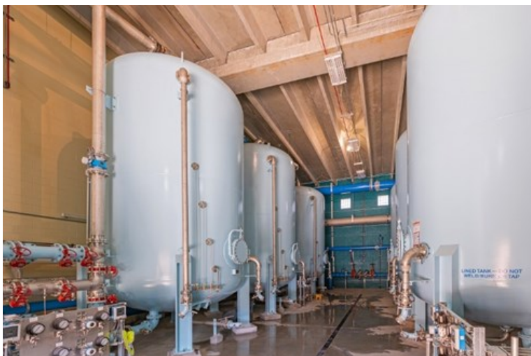
Eight new treatment tanks filled with granular activated carbon
