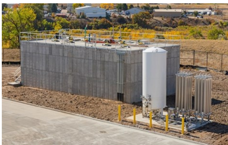
White Liquid Oxygen tank for ozone generation and concrete solids settling tank in background.
