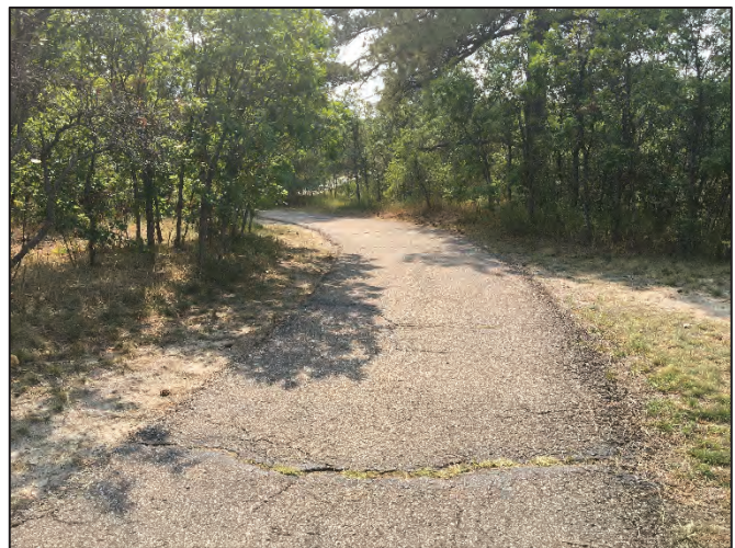
Photo showing current deteriorating conditions of asphalt section of trail in Woodlands Bowl Open Space.
