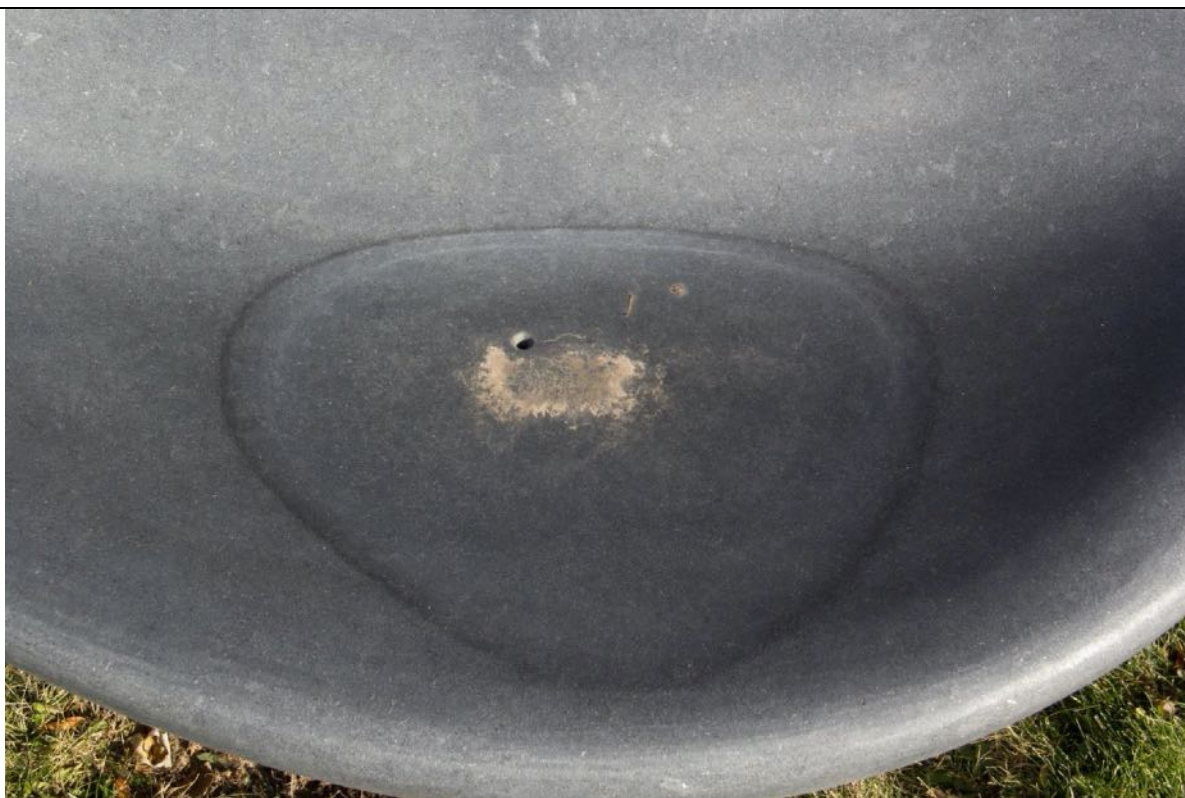
Detail: East bench seat with soil near drainage outlet and water staining
