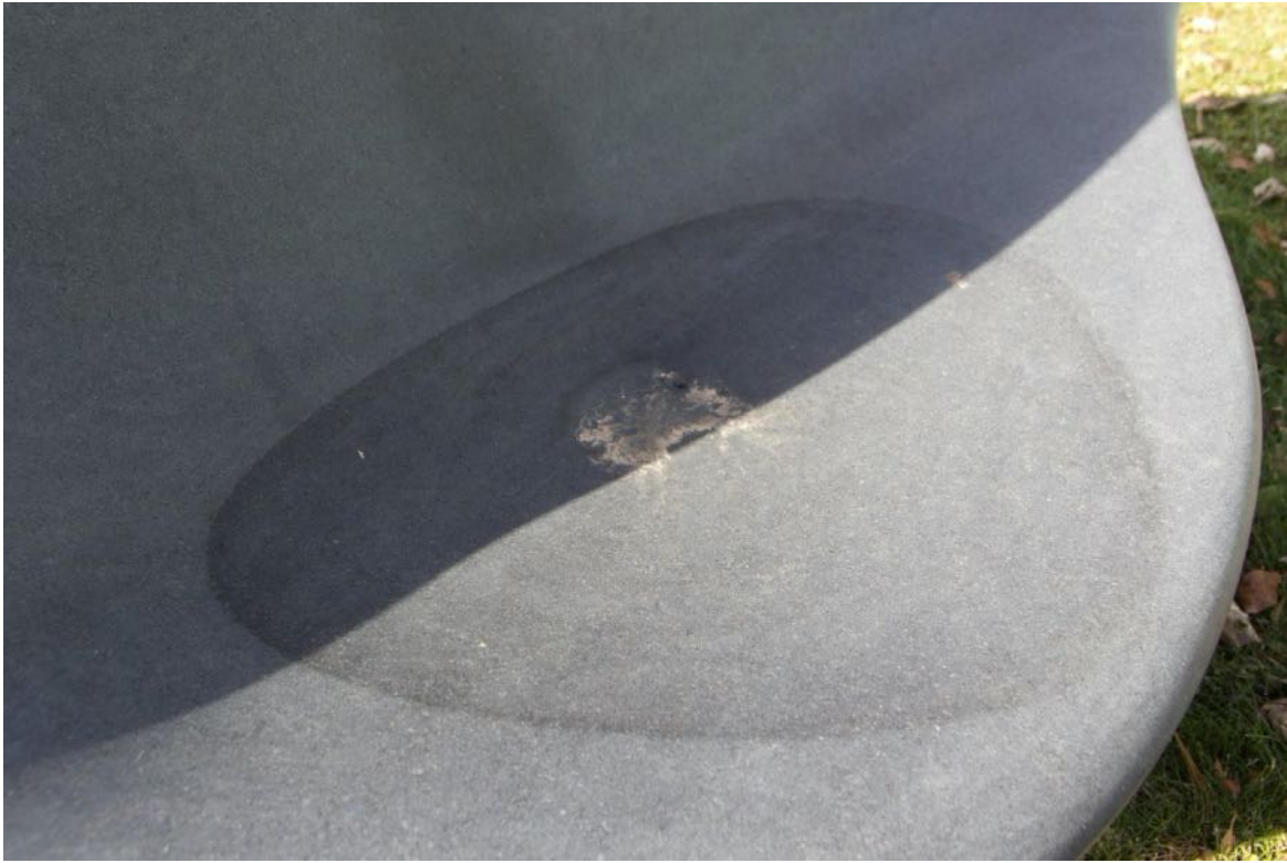
Detail: West bench seat with soil near drainage outlet and water staining
