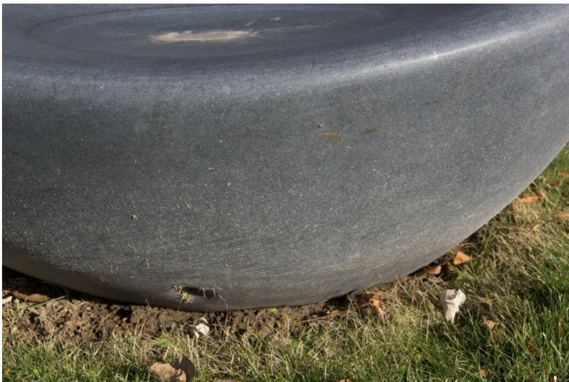
Detail: East bench front with surface soiling
