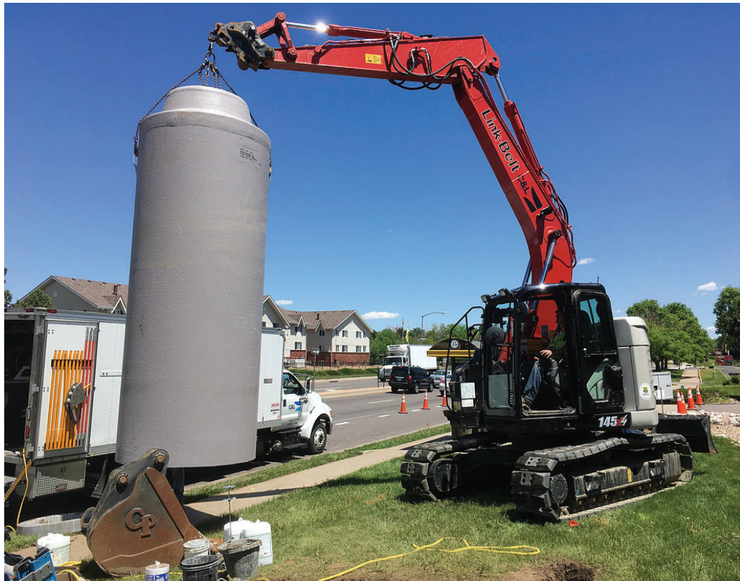
Manhole Replacement
