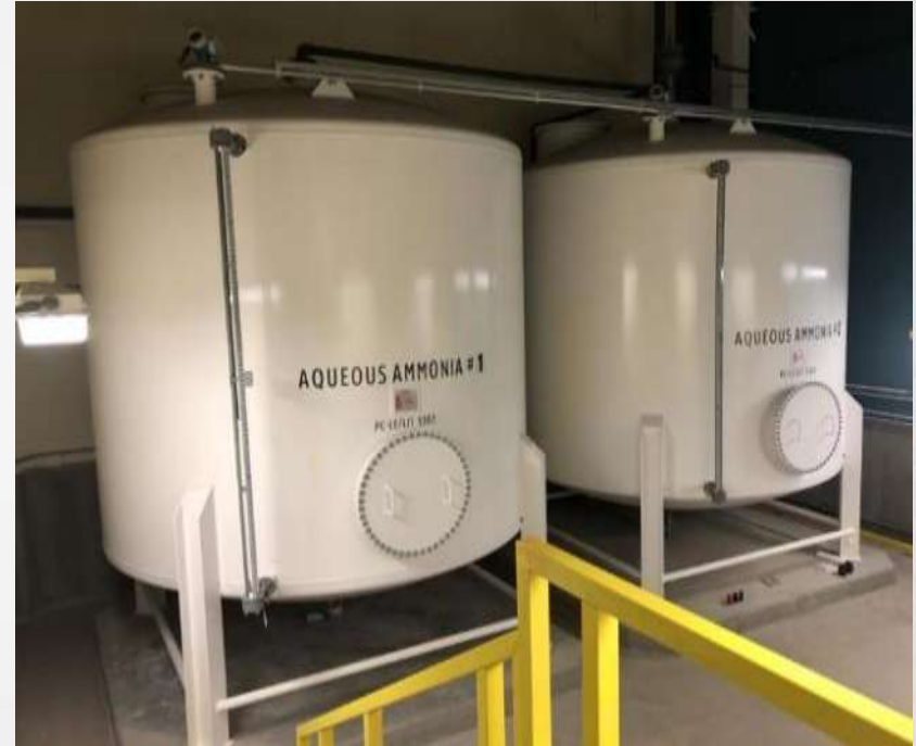
Ammonium Hydroxide Storage Tanks
