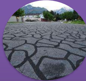
Crack Seal
