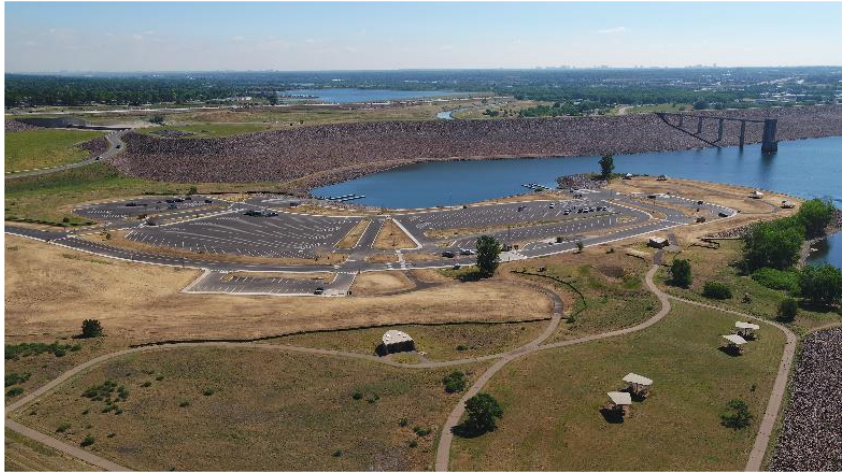
Reconstructed North Boat Ramp area
