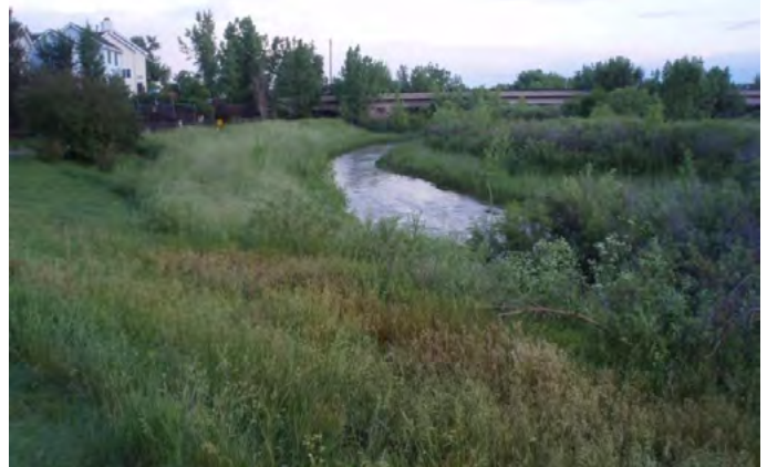
Before and after bank protection installation
