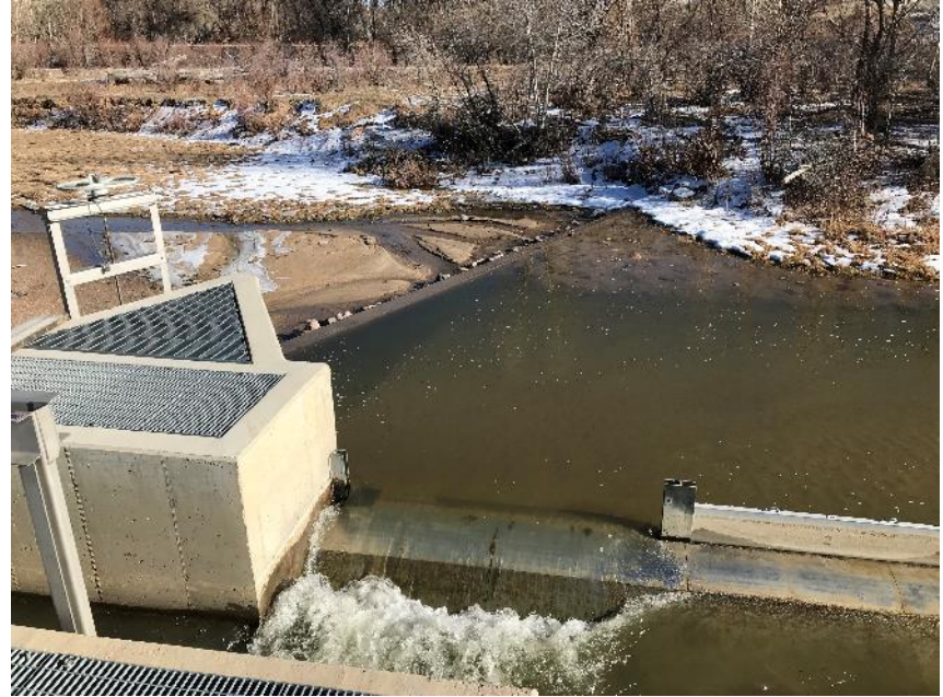
Plum Creek Diversion with gate 1 removed to allow water to flow into the infiltration gallery in January 2019.
