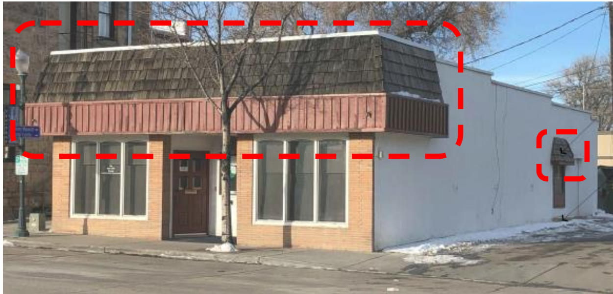
Cap Flashing, Mansard Roof, and Wood to be Removed, Highlighted Above
