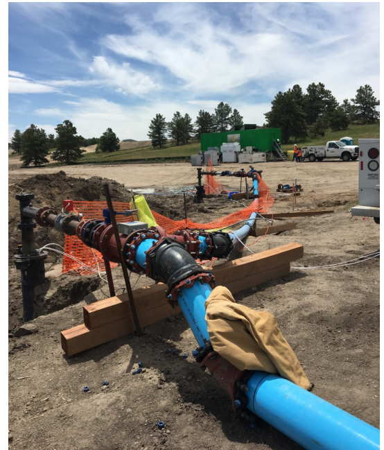
Temporary piping for the wells to run.
