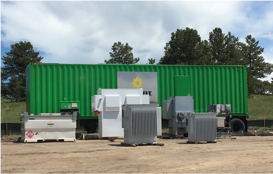
Temporary generator for running the wells.
