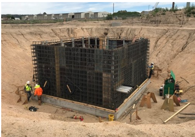
Steel wall reinforcing installed for raw water meter vault
