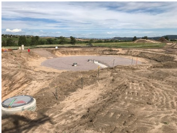
Base pad prepared for 1 MG raw water blending tank
