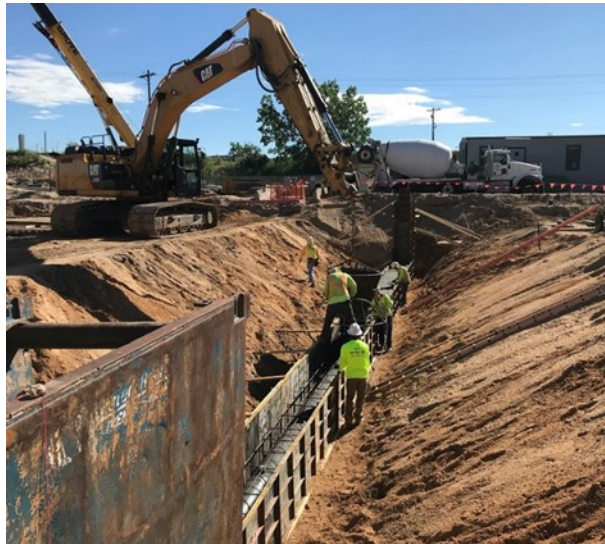
12-inch diameter water supply piping to new building being concrete encased
