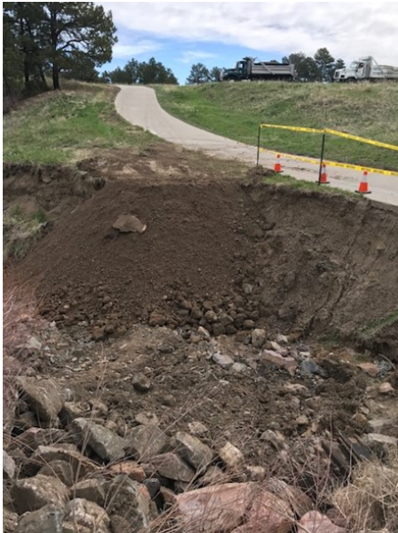
Area of erosion on top of the sanitary sewer line, adjacent to the walking trail, in The Meadows off of Sabercat. Repair, backfill, and prep work consisted of grading, resurfacing and rock placement for erosion control.
