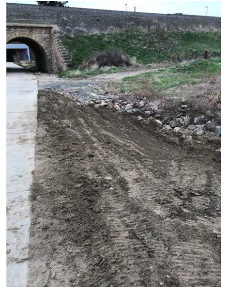
Area of erosion on top of the sanitary sewer line, adjacent to the walking trail, in The Meadows off of Sabercat. Repair, backfill, and prep work consisted of grading, resurfacing and rock placement for erosion control.
