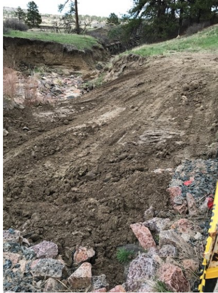
Area of erosion on top of the sanitary sewer line, adjacent to the walking trail, in The Meadows off of Sabercat. Repair, backfill, and prep work consisted of grading, resurfacing and rock placement for erosion control.
