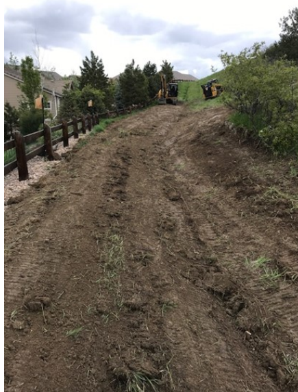
Renovation of the drainage swale behind the properties on Gould Circle.
