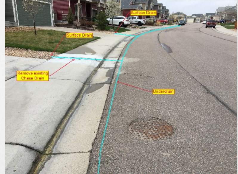
Subsurface Drain retrofit layout in impacted street
