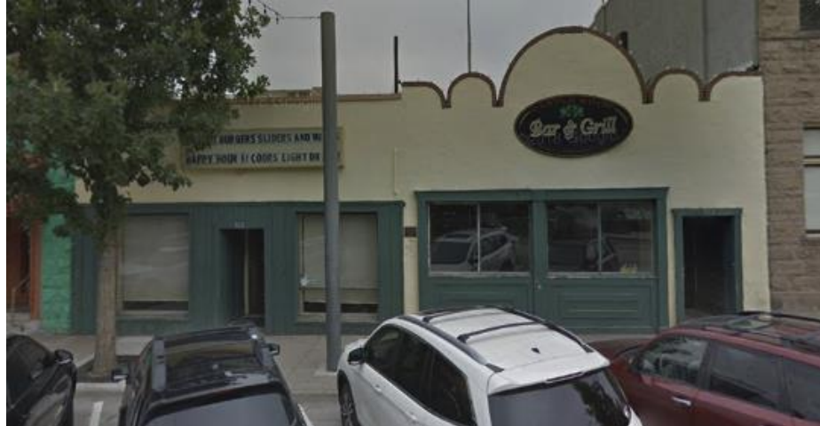
Street View of Existing Wilcox Street Façade
