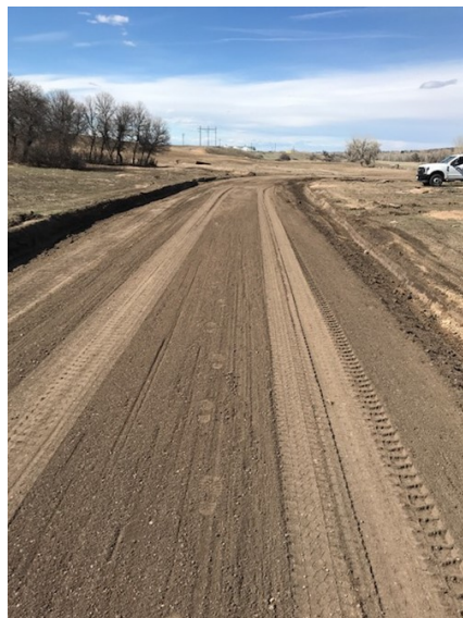
The Stormwater team restored the Plum Creek Diversion Pump Station access road. The quarter mile road was regraded, roadside ditches were cut in, and resurfaced with crushed concrete, making it safe and accessible in all weather.
