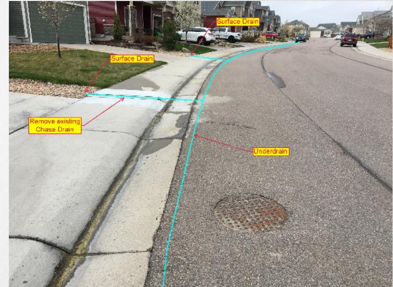
Subsurface Drain retrofit layout in impacted street
