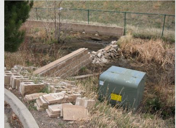
Pond Wall Collapsed due to poor maintenance
