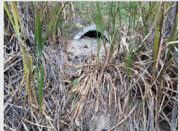
Sediment accumulation due to lack of maintenance
