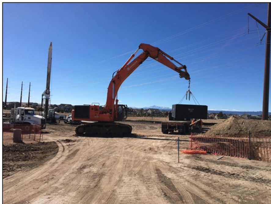
Setting a Vault for the Pipeline
