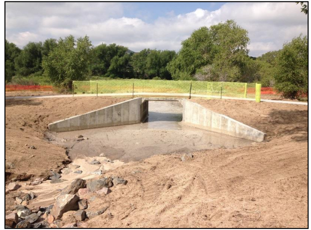
After: 10'x6' Box culvert at the East Plum Creek Trail
