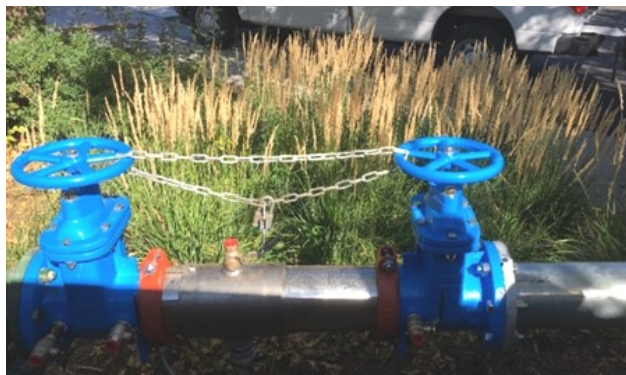
New 6-inch backflow in place
