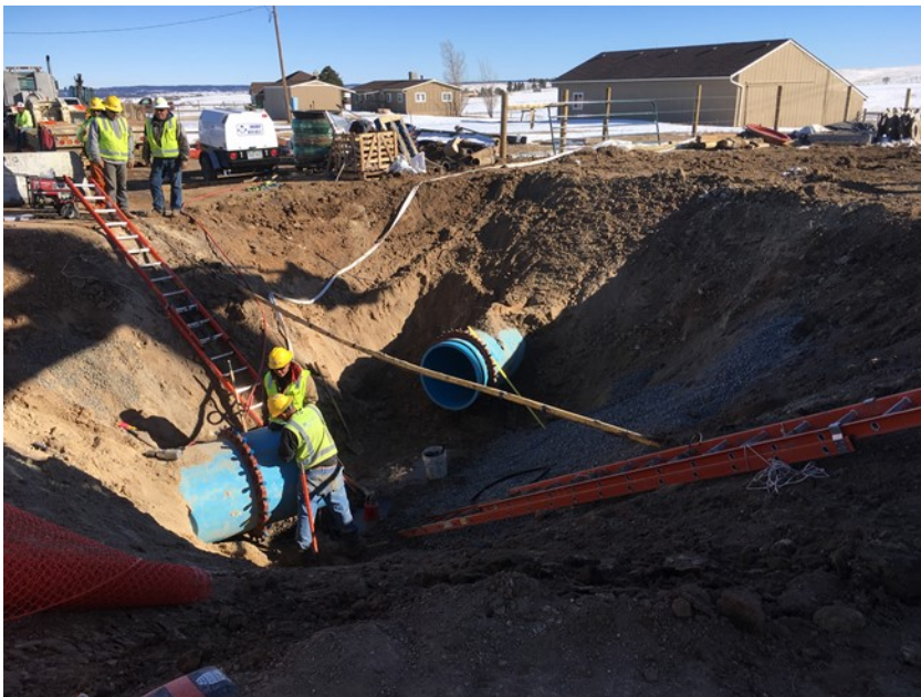
The final WISE piping connection was made to the PW&SD infrastructure at Outer Marker Road early in 2018
