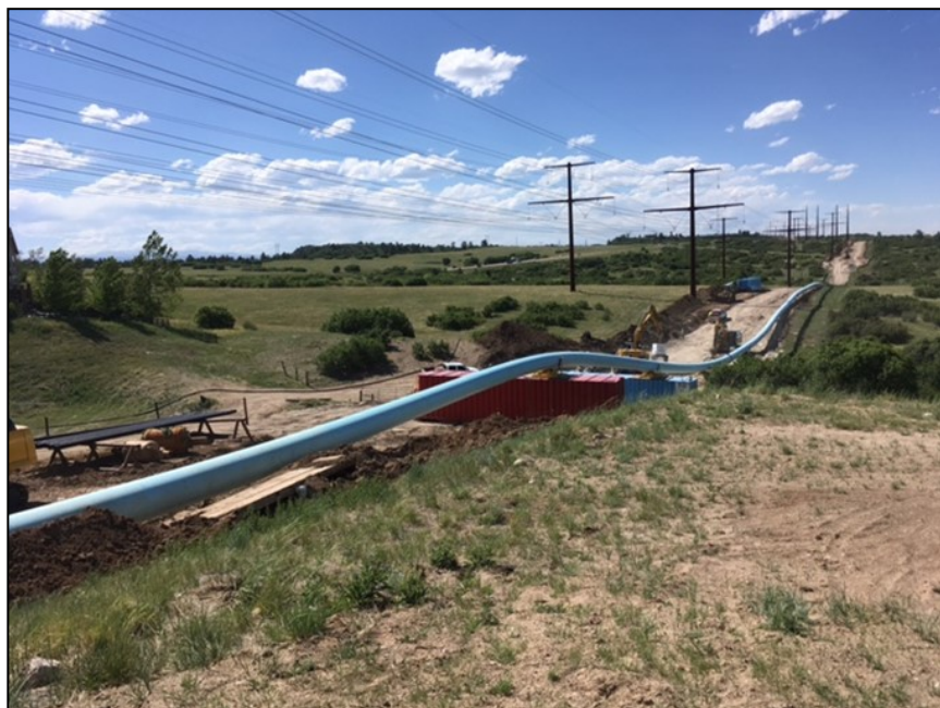
The WISE Pipeline during Construction
