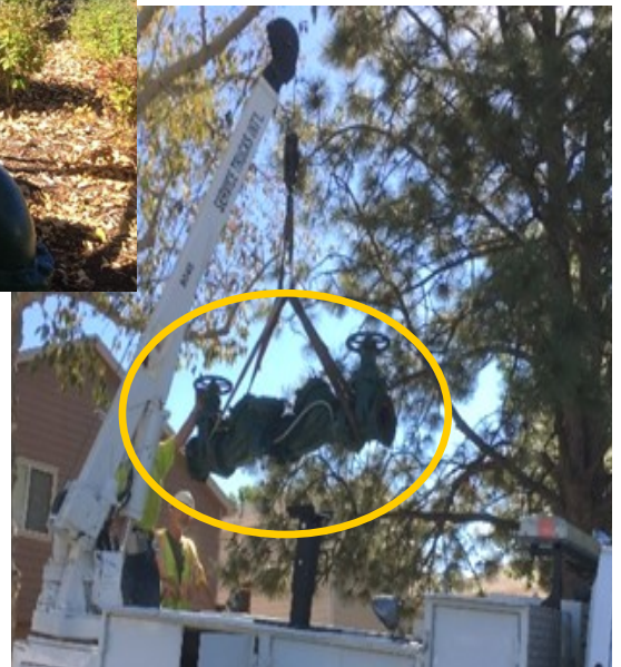
Removal of the 6-inch backflow
