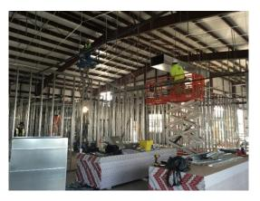
trim pieces on the outside of the building. Next month, the trim will be completed and the garage doors installed. Inside the building, the concrete floor was placed, which allowed interior framing to commence. Plumbers and electricians followed behind the framing to install pipes and wires in the walls.
