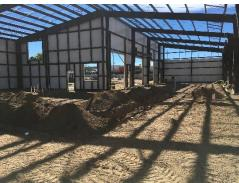
Inside the building plumbers worked on the underground plumbing for the maintenance bays, restrooms and break rooms, while electricians ran conduits to the main electrical distribution room.
