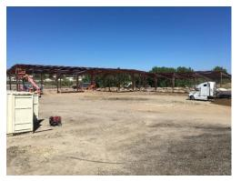
The project's general contractor, Taylor Kohrs, erected the steel structure. The siding and roofing panels arrived on site and will soon be installed. The structural soil import, site grading and underground utility installation also continued throughout the month.
