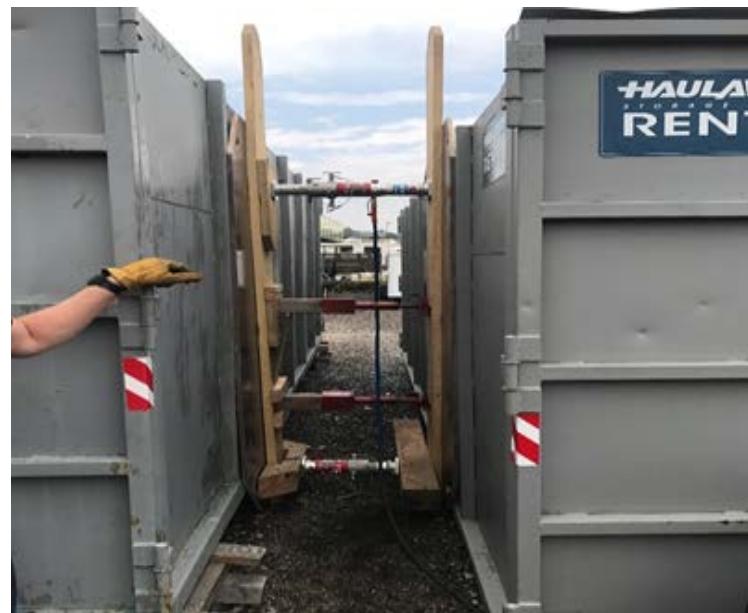
Members participating in Trench Rescue Operations Training - Ground Pads and Shoring
