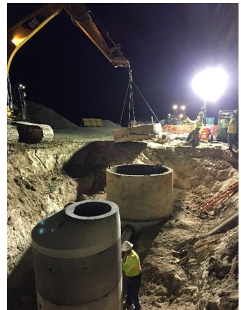
Maher manhole replacement at night
