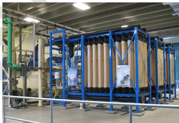
The membrane filtration system within the Plum Creek Water Purification Facility provides robust treatment through state-of-the-art technology.
