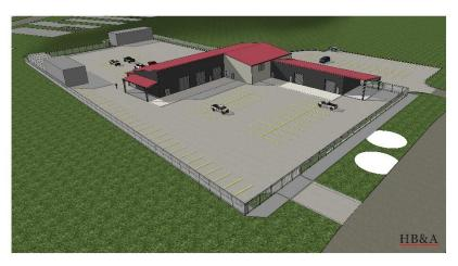
treatment plant. Building plans include five maintenance bays, indoor storage, a training facility, office space, a break room and a storage yard for equipment and material.
