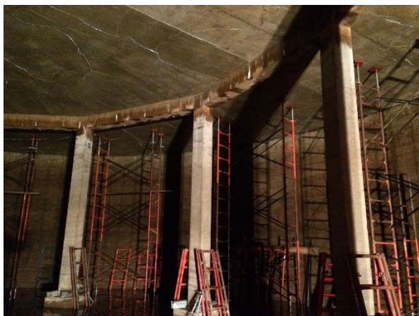
Temporary Shoring Inside Tank 3
