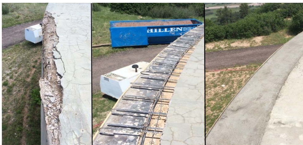
Tank 3 Concrete Roof Repair Sequence
