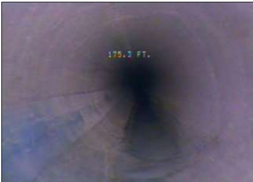
Post CIPP: Pipe after rehab with cured in place pipe; the liner seals cracks and joints and eliminates I/I and future root intrusion.
