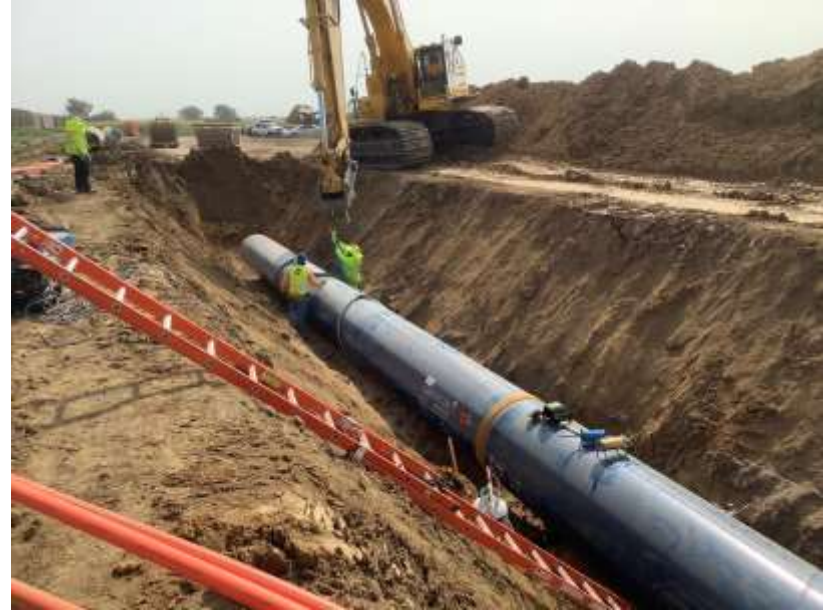
A recent B&McD project using 42" diameter welded steel waterline in Thornton, CO
