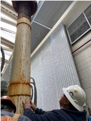
Removal of a Ray Waterman Green Zone Pump
