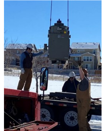
Ray Waterman Green Zone Pump Motor and motor removal
