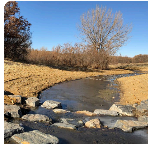
Boulder cascade and riffle sequence on McMurdo Gulch Priority 1.
