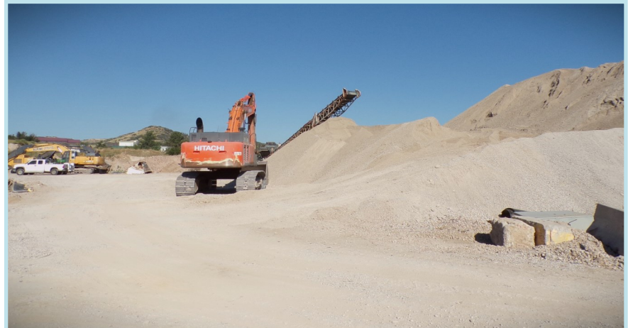
Demolition for the future Brickyard site.
