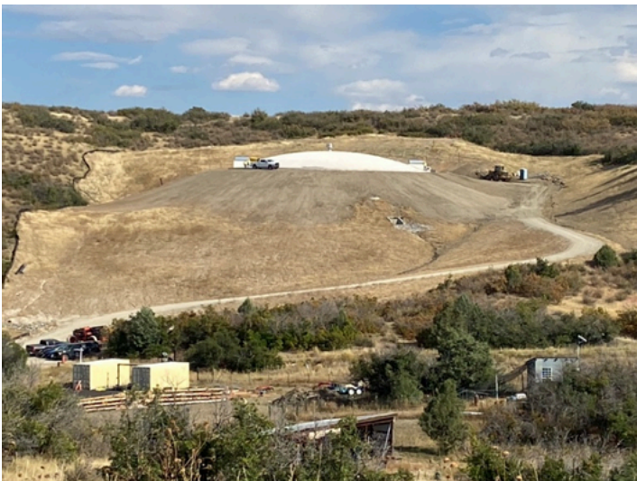
Tank 18 dome peaks from sub-terranean site.
