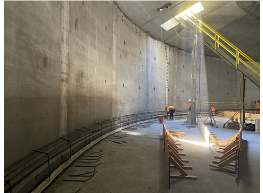
Contractors working on repairs inside Tank 18
