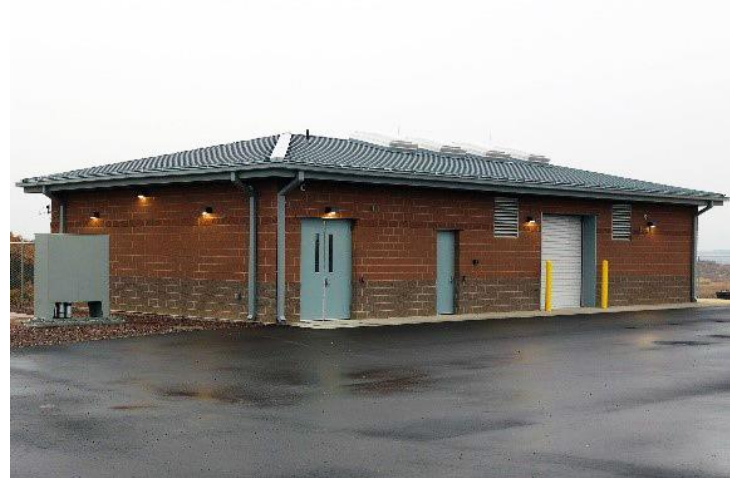
PWSD's Canyons Pump Station used to deliver flows from Pressure Zone 2 to PZ 3
