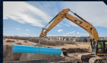
36-inch PVC pipe has a long service life and is unaffected by overhead transmission lines and highly corrosive soils.
