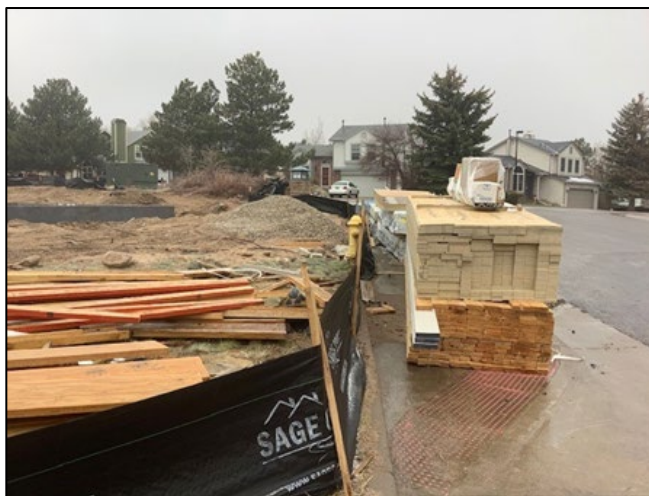
Hydrant blocked by construction materials placed on sidewalks in a development with occupied home.
