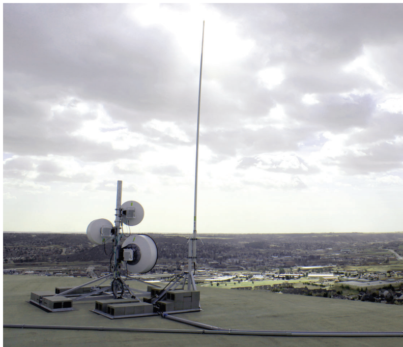
▲ Advanced Metering Infrastructure (AMI) antenna
