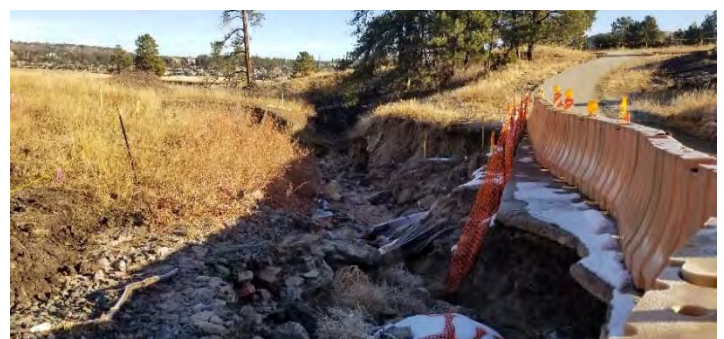
Figure 3 - Collapsed Trail and Eroded Stream
