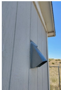
Venting of chemical storage tank
