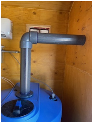
Venting of chemical storage tank
