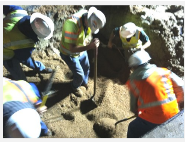
The team, working at night, to fix a leak.
