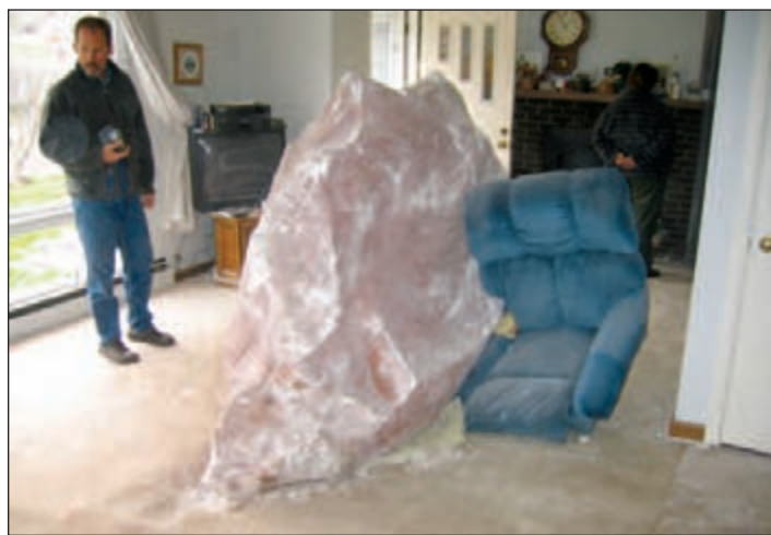
Figure B: In April 2004, this rock from the source area shown above smashed through the wall of a home and came to rest against an easy chair. The homeowner built a rockfall protection fence afterwards. (Photo taken in 2004 by Steve Vanderleest, City of Glenwood Springs.)
