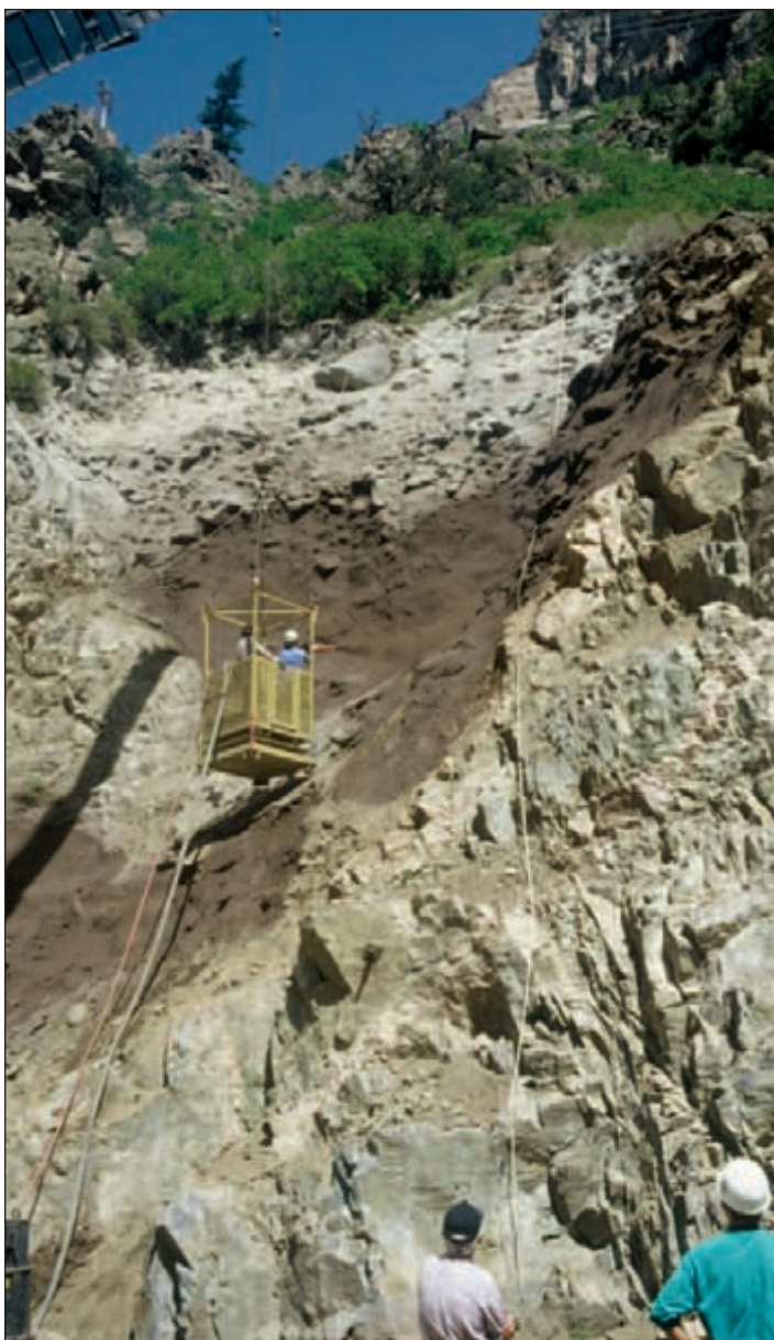
Figure 15: Application of shotcrete at a raveling cut-slope exposed in a rocky talus chute. The concrete has been dyed dark brown to better match the surrounding area. (Photo by Jon White.)
