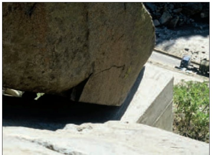
Figure 14: Smaller, upslope concrete buttresses are anchored to the rock face with rockbolts. Then, concrete rebar and wood forms are wired to the anchors in Glenwood Canyon. The concrete is carried in mud buckets by helicopter. The three photos show the progression of the installation. (Photos by Jon White.)
