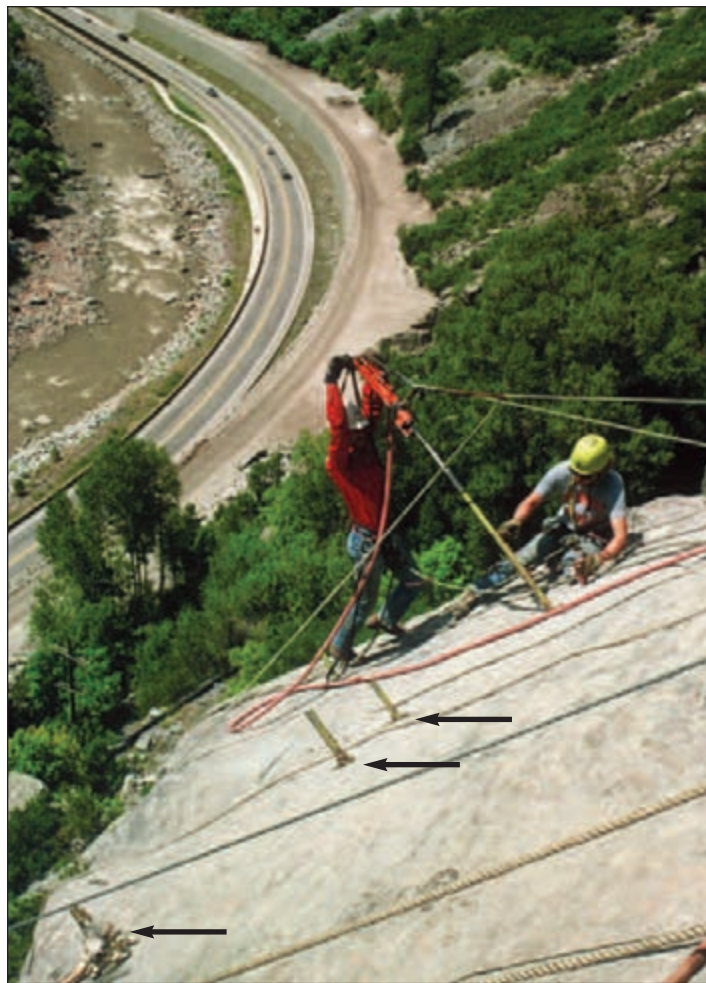
Figure 12: Installation of rockbolts on the rocky slope of Glenwood Canyon during the Interstate 70 highway construction project in 1991. The worker is spinning an epoxy-coated steel bar into the drill hole using a pneumatic drill. The protruding bars in the foreground (shown by arrows) are installed rockbolts. (Photo by Jon White.)
