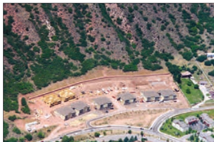
Figure C: This newer development in west Glenwood Springs constructed a rockfall impact wall above their townhomes to protect against both rockfall and mudslides (debris flows). (Photo by Jon White.)
