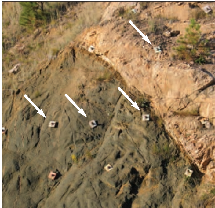
Figure 13: Pattern rock bolting to reinforce the rock cut along Highway 285. The threaded steel bars have been cemented into drill holes. The external evidence of rock reinforcement is shown by the steel plates and large nuts, four of which are indicated with arrows. (Photo by TC Wait.)
