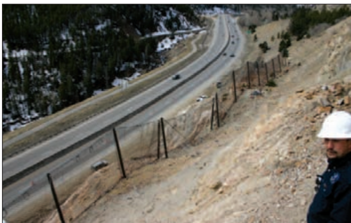
Figure 11: Wire rope rockfall fence installed on a rock slope at Georgetown Hill above Interstate 70. Exit ramps shown in the upper part of the photo are for the Silver Plume Exit. (Photo courtesy of Ty Ortiz, CDOT.)
