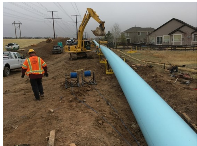
Fused pipeline being pulled towards lower right and through the HDD hole.
