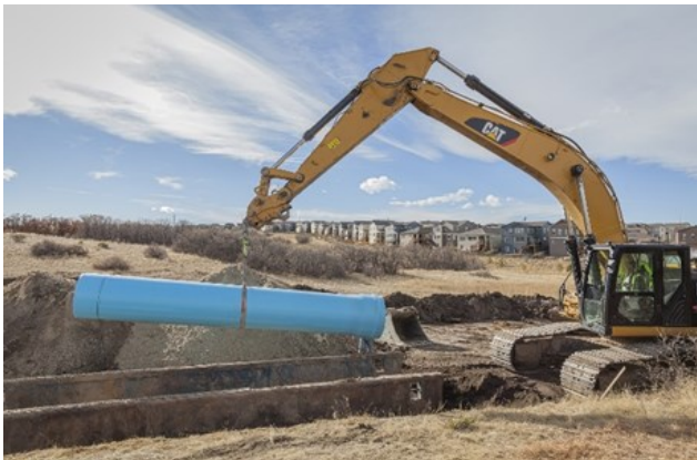
Typical 36" diameter pipeline with push-on joint connections being lowered into trench.
