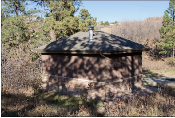
Figure 18: Natural fuels surrounding a pump station
