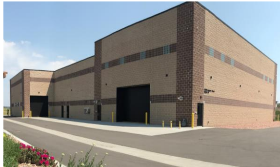
Advanced Treatment Building
