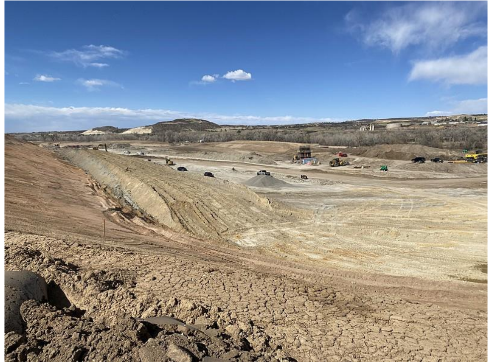
Construction of CRR2
