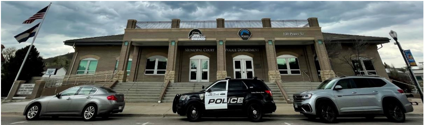
Castle Rock Police Building
