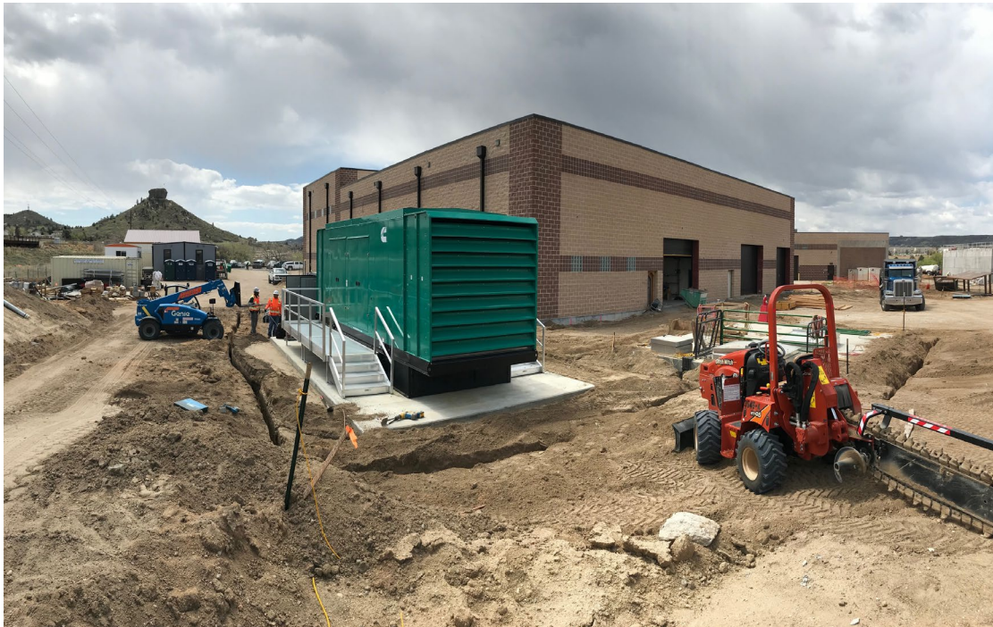
Advanced Treatment Building
